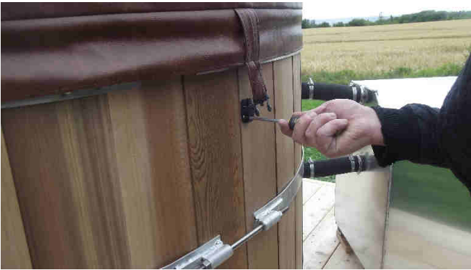
Fig. 10.4.1 Attaching the cover strap buckle.
