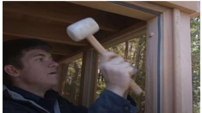
Install the door handle by placing the provided 2" (50mm) lag screws through the inner handle (short) into the outer handle (longer)
