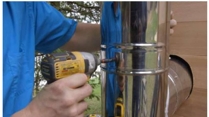
Wrap the chimney support strap around chimney and use the provided nut and bolt to secure.
