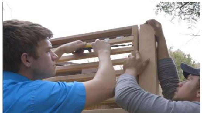
Install the door plugs by pushing them into the pre drilled holes then tapping them in tight with a rubber mallet.
