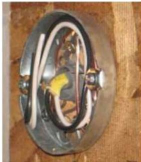
Recommend low profile "pancake box" rather than standard octagon box. This can be surface mounted flush inside of the sauna with light fixture fitting over the box.
