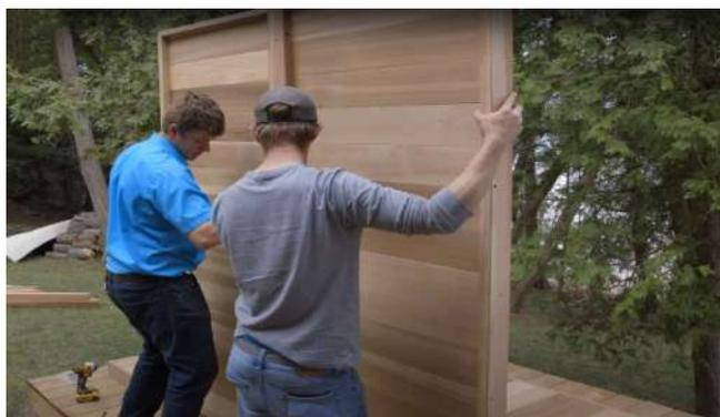
Connect the wall panels together using 2 ¾" (70mm) connector bolts and a connector cap nut. Using the provided hex keys, snug up all the bolts.
