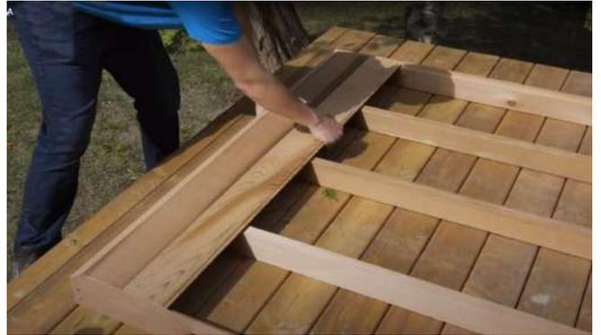
Fasten the floor boards into the floor joists and the inner floor joists with 1 ½" (38mm) screws.
