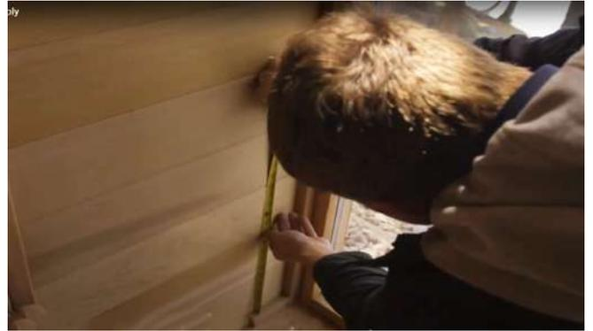
Install the supplied support screws into your marks as shown. Screw them in until they are about ¼" (6mm) out of the wall.
