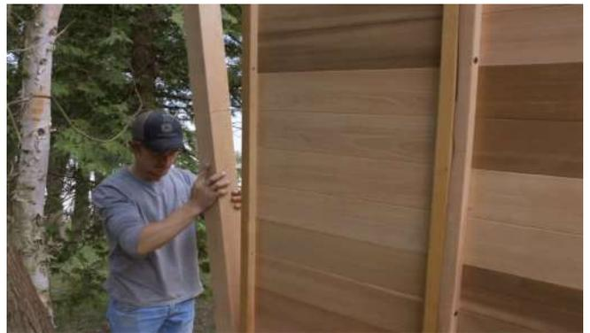
Position the walls onto the base ensuring there is 1 ½" (38mm) overhang on each side.
