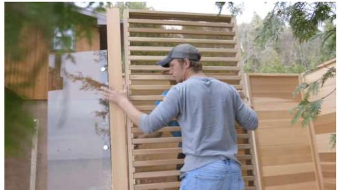
Make sure the next window panel is flush to the first one and fasten it together with 2 3/4" (70mm) connector bolts and a connector cap nut.
