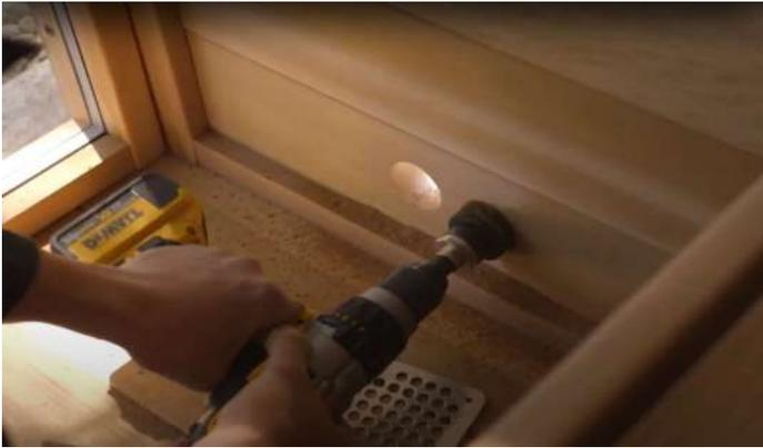
If an electric heater is chosen, Drill inlet holes centered under the heater close to the floor.
