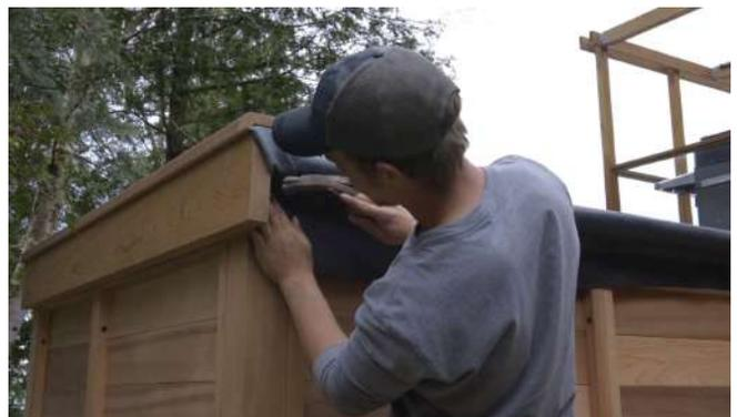
Place the back trim piece up tight under the edge of the roof.
