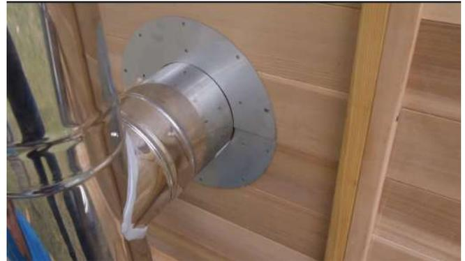
Attach the rain guard to top chimney piece and secure with provided screws.
