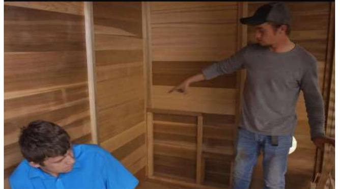
Ensure the bench supports are tight to the side and back walls, then secure the supports to the walls and floor using 2 ½" (64mm) screws. Repeat on other end.
