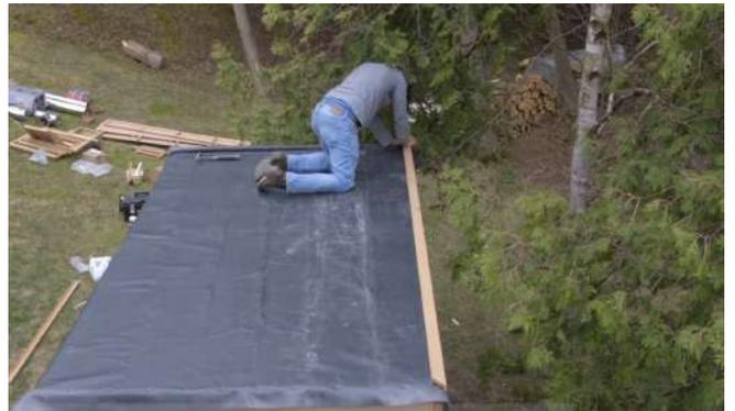
Line up the roof cap pieces so the corners are tight together and tap them down tightly over the trim pieces with a rubber mallet.
