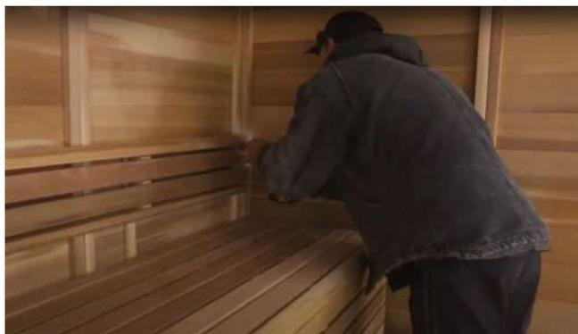
You can now secure the lower front bench enclosure to the bench supports by screwing between the slats using 2 ½" (64mm) screws.
