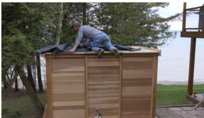
Once the membrane is laid out evenly over the top of the sauna, use staples or nails to secure it to the trim pieces.
