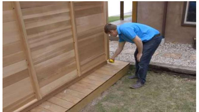
Once the sauna walls are overhanging 1 ½" (38mm) on all sides of the floor, use 2 ½" (64mm) screws to secure to the base through the pre drilled holes.
