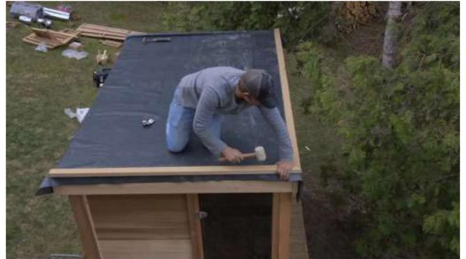
Using the supplied finishing nails, secure the roof caps into place.
