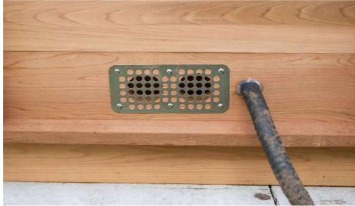
Install 1 of the stainless steel vent grills over the inlet holes on the outside of the sauna centered over the holes using 1 ½" screws. (38mm) (6pcs)
