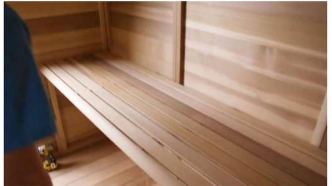
Line up the remaining bench supports with the braces on the bottom of the top bench.
