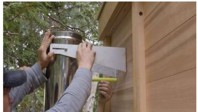
Tighten up the chimney support brackets with a 7/16" (11mm) socket or wrench until snug.
