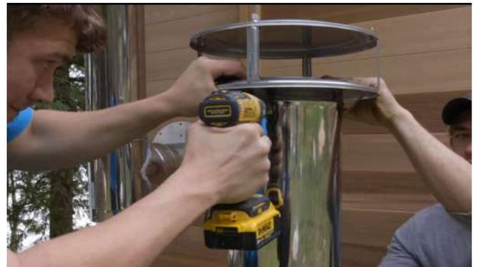
Attach chimney top onto the chimney and secure them together with the provided screws.
