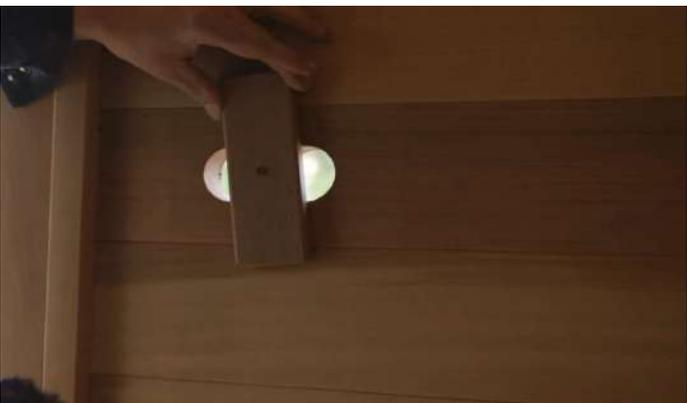
Install the cedar vent cover over the outlet holes on the inside of the sauna with a 1 ½" screw.
