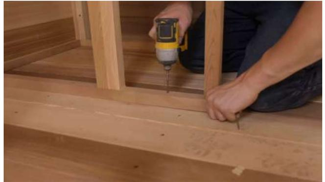
Secure the bench supports to the top bench from underneath using 2 ½" (64mm) screws.
