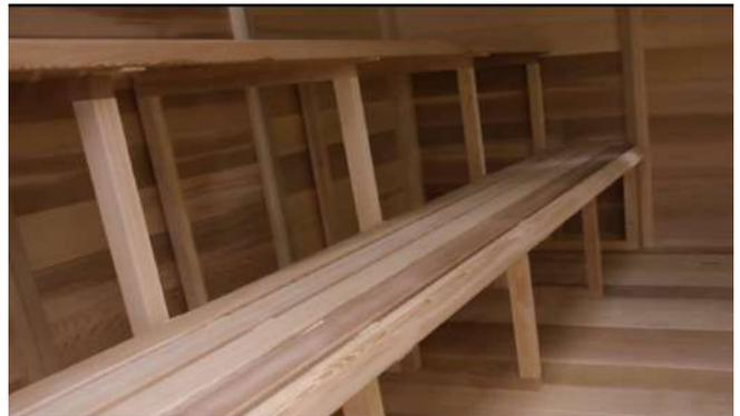
Secure the bench supports to the bottom bench from underneath using 2 ½" (64mm) screws.
