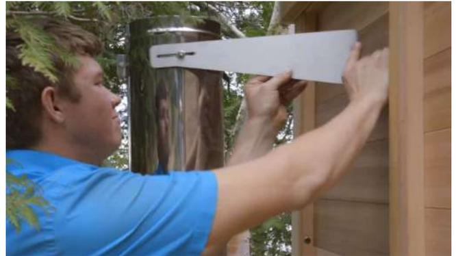
With the nuts on the side of the straps loose, level up the chimney pipe.
