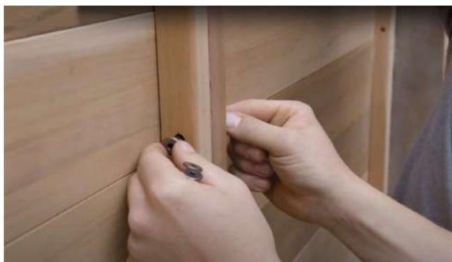
\* Note that the walls should be assembled so the bolts should be on the outside of the sauna.
