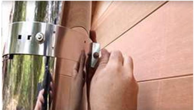
Attach chimney support braces to the support strap and thread the nuts on hand tight.
