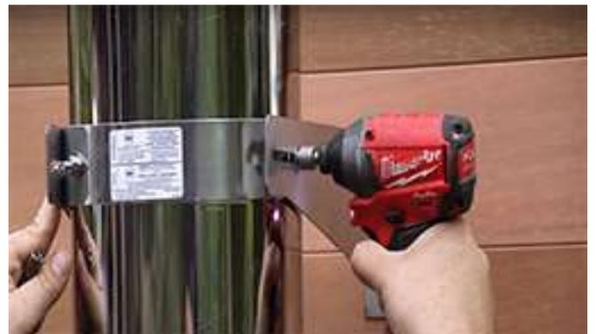
Attach the chimney cover plates starting with the bottom plate, using 1 ½" (38mm) screws ensuring the top plate overlaps the bottom and that they are level
