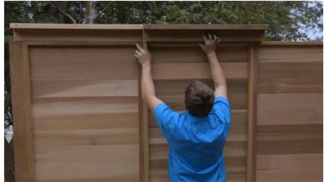
Inside , line up the holes and fasten the roof panels together with 2 ¾" (70mm) connector bolts and connector cap nuts.
