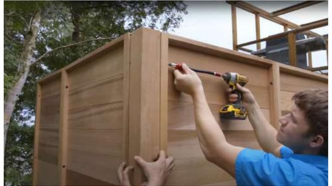
Secure the side wall to the post in the same manner ensuring that the outside of the wall is flush to the post.
