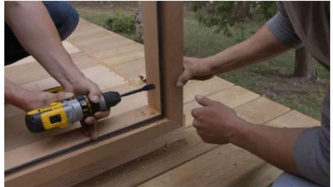
Secure the door frame to the last corner post using the 2 3/4" (70mm) Connector lag screws through the pre drilled holes.
