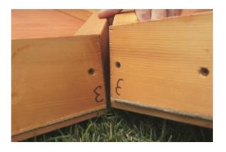
17. Secure 2 roof panels together using the supplied bolts, washers and nuts.
