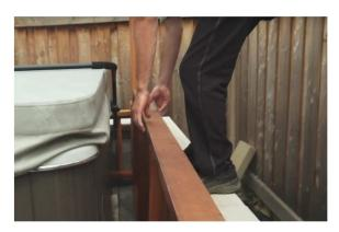
7. Secure lower side railing flush with opposite corner post using provided screws into pre drilled holes.
