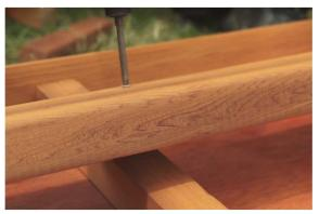
16. Take 2 roof panels at a time and line them up as shown. Make sure the numbers match where the roof panels connect.
