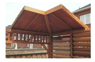
19. With bolts and nuts provided, secure roof panels together through pre drilled holes.
