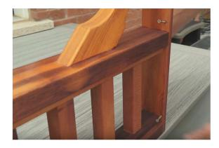
9.Starting between the two back posts, Line up top railing flush to top of posts and secure using provided screws.
