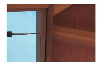
23. Secure top railings and walls to roof panels. Be sure to line up the screws so thay are fastening through to the roof joists.
