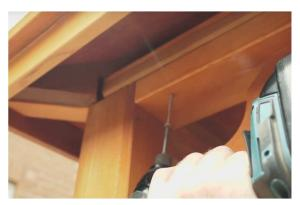
24. Pre place screws using the holes provided in the ridge cap and trim pieces for easier installation.
