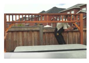
11.Line up shutter wall flush to post and sitting on top of solid bottom wall. Secure with provided screws.
